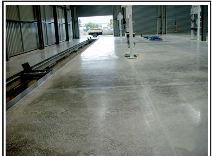
Caopower South Australia used Densi-Proof plus Surface Sheen at time of pour and virtually eliminated any cracking. They have a hardened surface that protects against oil, acid attack, and is attractive and easy to clean.
